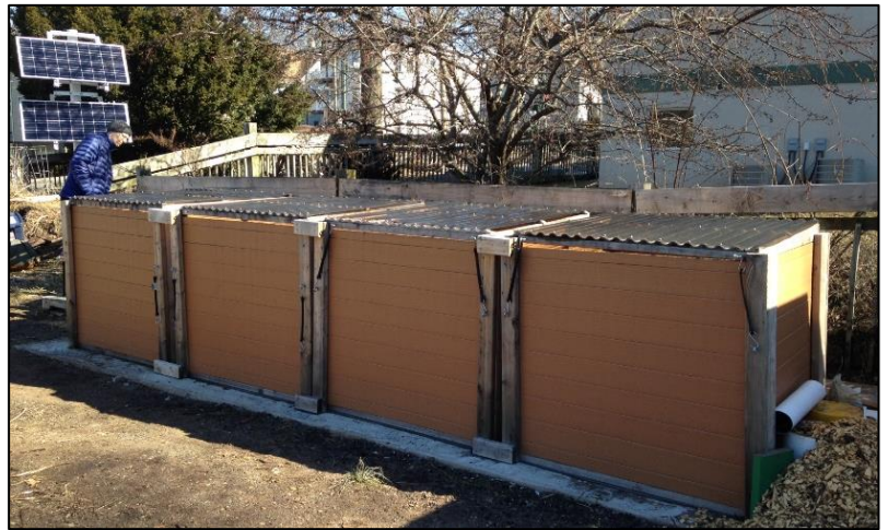
Finished four-bin aerated static compost bin system
